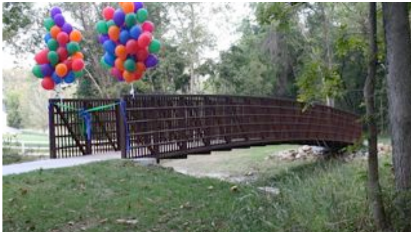
NOW: Today, Lantz's bridge stands strong at it's new home at Prairie Creek Trail in Platte County
